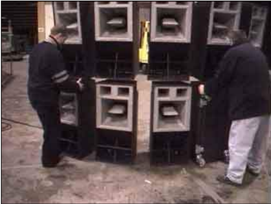
Fig 4.5-13 Raise the grid & move the next row of enclosures in place
