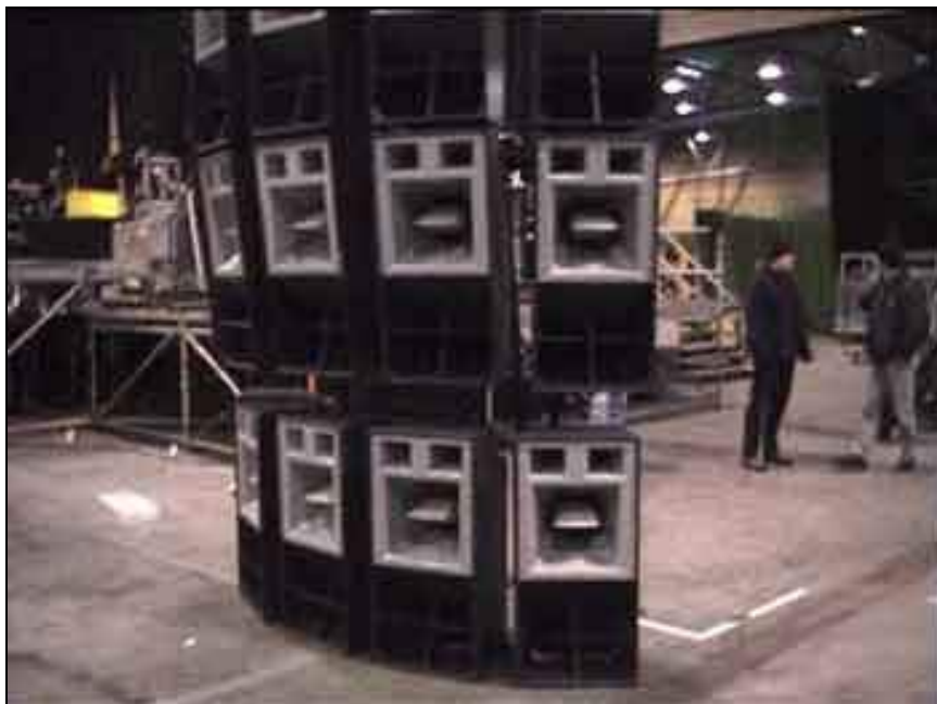
Fig 4.5-20 The array can then be raised again ready for the next row of Resolution enclosures
